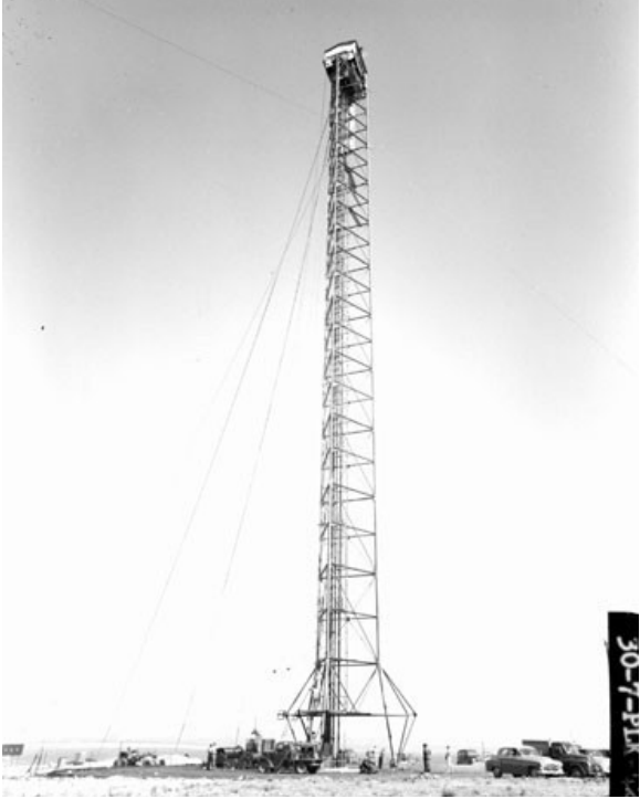
Tower T-4, Snapper #2 tower shot
